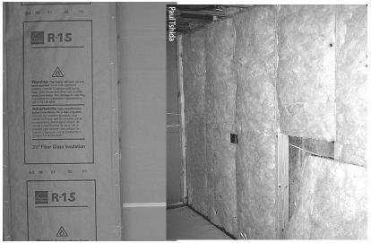
**R-15 fiberglass batts:** Install R-15 batts in open walls and attach them to the face of the stud as shown above. Or install unfaced batts as shown below. Either way, cut the batts accurately and install them carefully.
