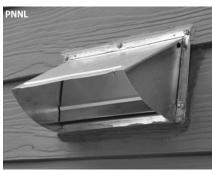
**Termination fitting:** If the fan operates intermittently, the termination fitting or the fan must have a backdraft damper.
