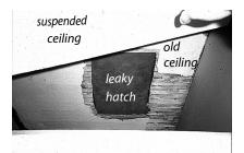
Sealing existing upper ceilings: With a non-structural suspended ceiling and a damaged plaster ceiling above, seal the plaster ceiling above if it's impractical to air seal the suspended ceiling.
