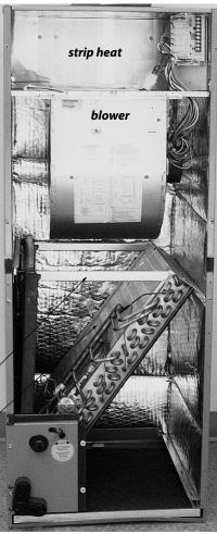
**Heat pump:** This upflow indoor air handler contains a blower, indoor coil, strip heat, and filter bracket.
