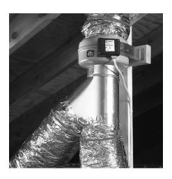
In-line fan in attic: A Y guides exhaust airflow from two bathrooms for both local exhaust and whole-building ventilation.
