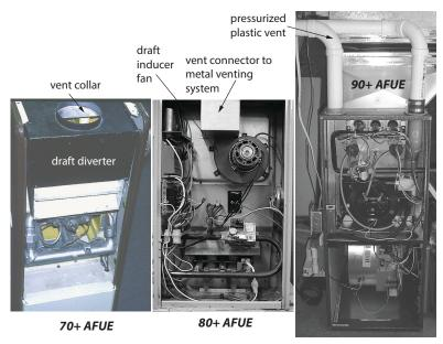
**Gas furnace evolution:** Energy auditors should be able to identify the 3 types of gas and propane furnaces. Only the 90+ AFUE furnace has a pressurized vent. The two earlier models vent into traditional atmospheric chimneys.
