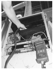
**70+ Furnace:** Sample flue gases within the draft diverter inside each exhaust port.
