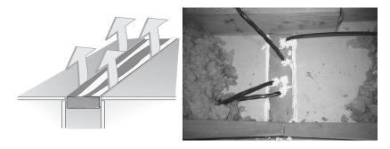
**Leaky top plates:** The cracks along top plates are from lumber shrinkage. They are small cracks but there are long lengths of them.
