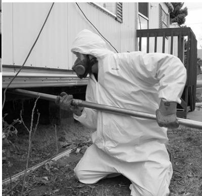
The preferred method is to spray foam the belly, using high density spray polyurethane foam (SPF). It is applied at a 3-inch thickness and is a continuous application.
