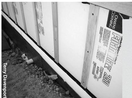
**Foam sheathing with battens:** One-by-four battens are applied to 4 inches of foam board on the exterior provide a fastening strip for siding and trim.
